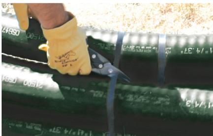
1 - Cut the three outermost fixing bands.
